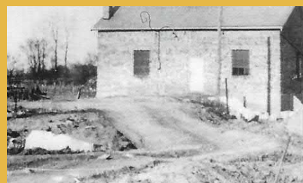
Andrew Kroeger slaughterhouse built in 1927. It was renovated by sculptor Don F. Wiegand for his studio in 1965. Courtesy of Don Wiegand.
